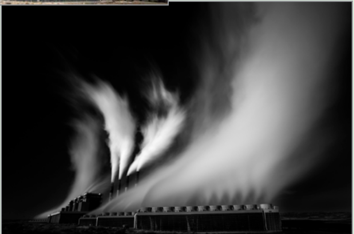
Jim Bridger Power Plant - After © Cole Thompson
